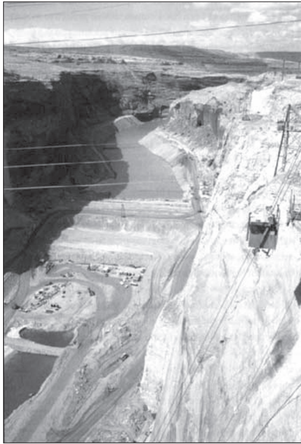
Figure 3 — Photographs of Glen Canyon Dam under construction, Lake Powell is behind
